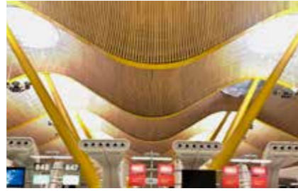
Madrid Barajas Airport
